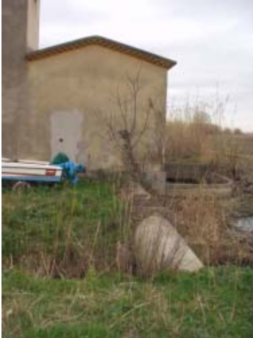
Station de pompage
