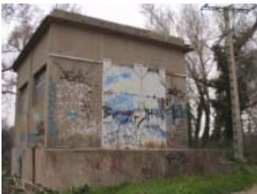
Station de pompage
